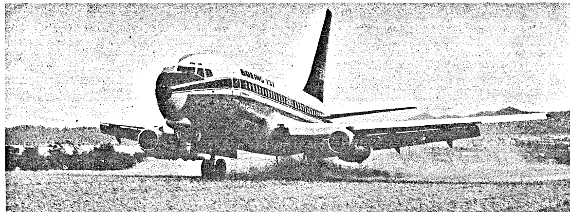
A Boeing twinjet recently made 25 landing/takeoff sequences on the secondary gravel runway at Lake Havasu City, Ariz., during final Federal Aviation Administration certification tests.
